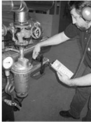
Figure A-14 Checking a steam trap with a Direct Contact probe
