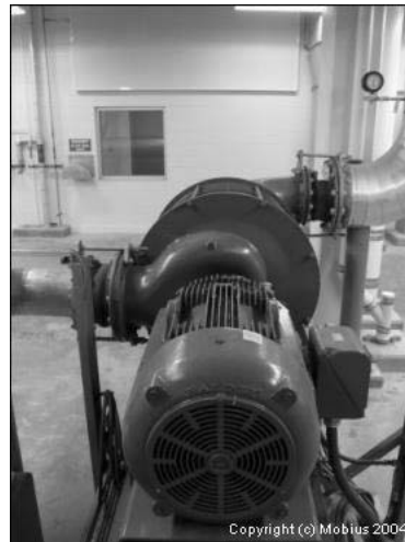
Figure 16-29 Compute thermal growth for larger machines
