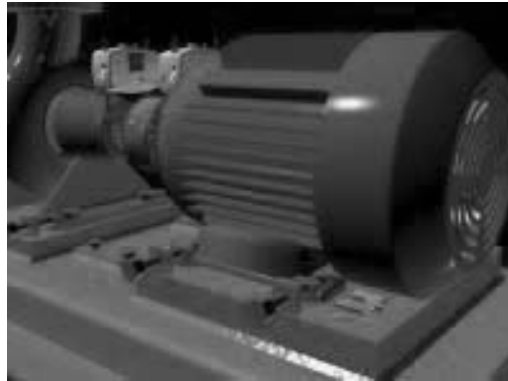
Figure 16-37 Checking for soft foot using a laser alignment system
