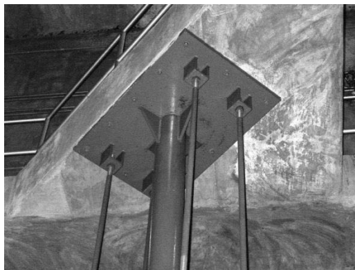
Figure 7-15 - Pipe Hanger Assembly Attached to 4th floor Beam
