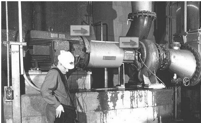
Figure 6-98 - Adjust axial readings for sensor direction
