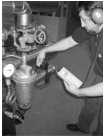
Figure 23-17 Checking a steam trap with a Direct Contact probe
