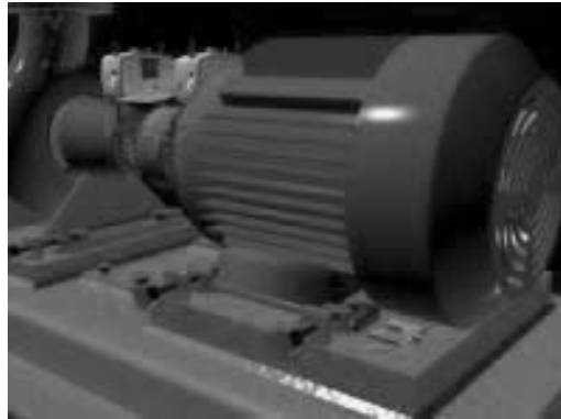
Figure 12-37 Checking for soft foot using a laser alignment system
