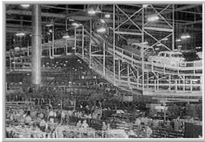
Figure 22-10 For many years the maintenance philosophy has been just to keep the plant running and deal with the failures when they occur.
